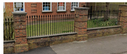
EXAMPLE OF PROPOSED FRONT BOUNDARY WALL WITH METAL RAILINGS - NATURAL SCREENING BEHIND
